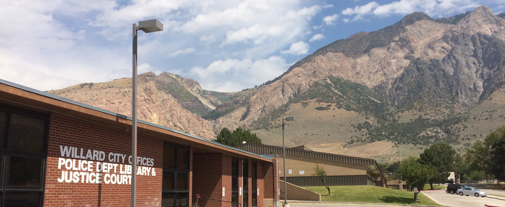
Willard City offices
