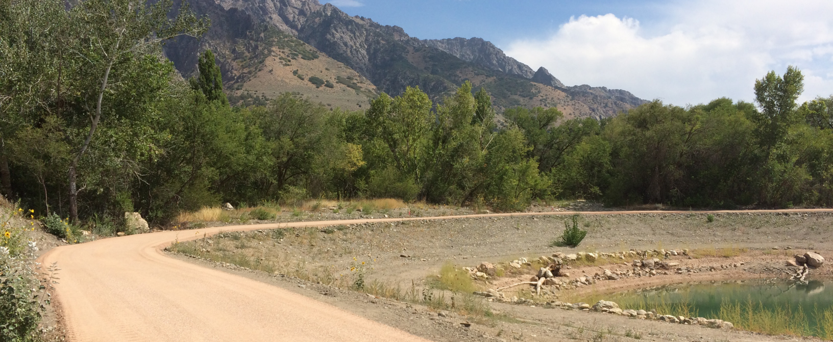
Construction of the Willard Creek Debris Basin Park & Pathway
