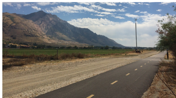
Figure 3-6. Existing section of the HOP located on the north end of Willard.
